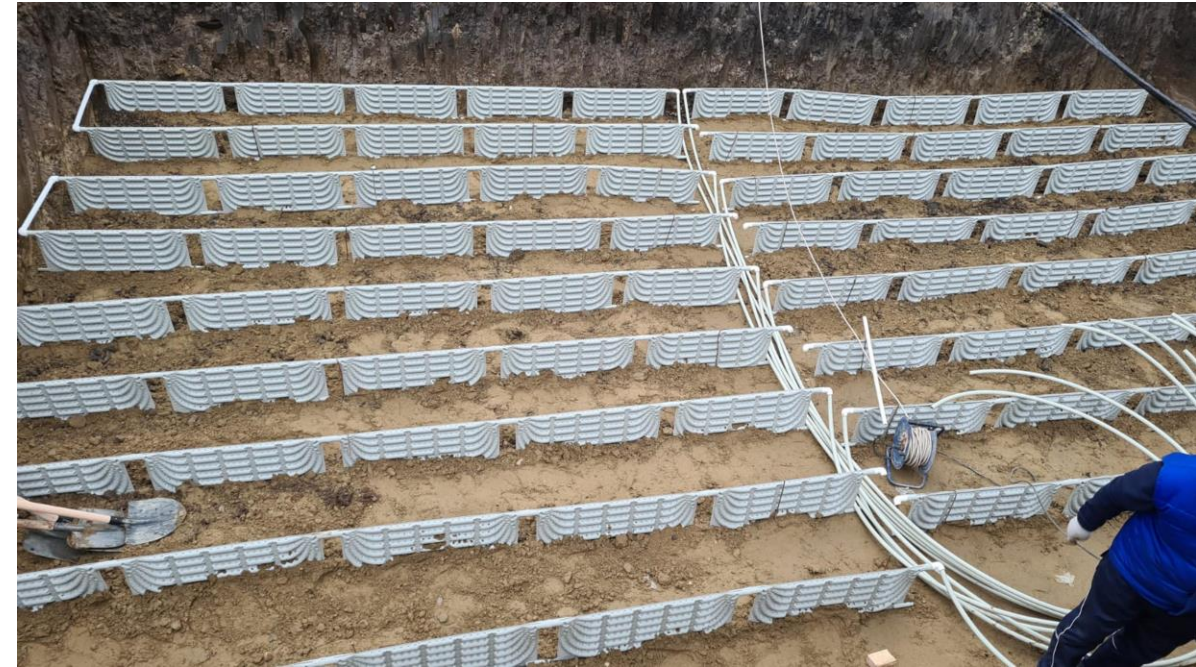
University UPG Piolesti campus: Georegisters for extraction of ground heat. Innovation Norway Grants
